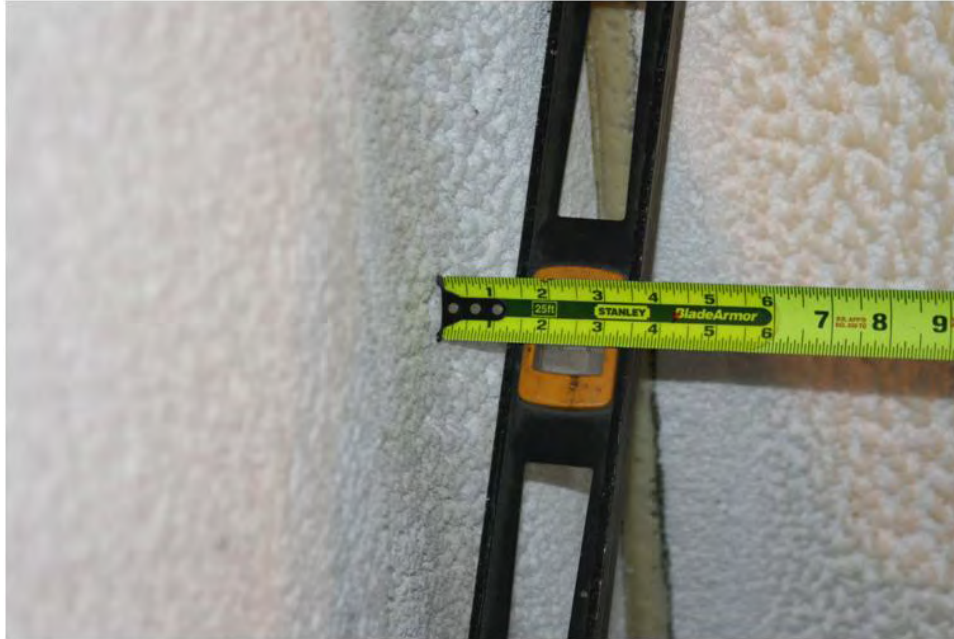
Figure 7. Back Wall: Post-Test View without Metal Sheeting. Nominal 1 3/8-in. Melting Depth at Crib Corner.
