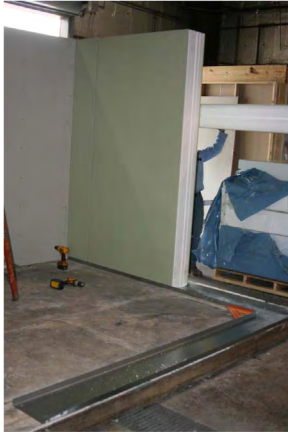
Figure 9. Open C Channel and Test Wall Construction.
