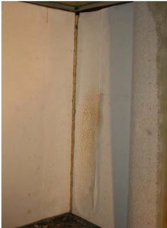
Figure 6. Post-Test View without Metal Sheeting.
